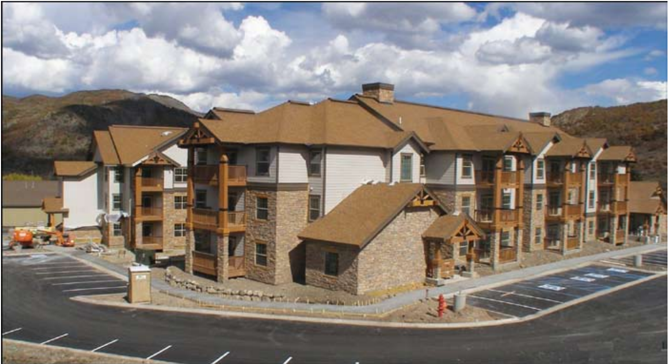
Shown only weeks before its opening, the Club Commons II will house more than 120 employees of the Aspen Skiing Company just in time for the winter season. The entire 44,000 sq. ft. complex is built to LEED certification.
